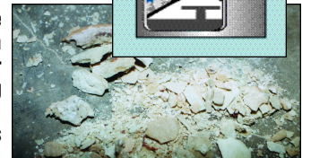
Scale Removed from a Hot Water Plumbing and Heating Systems
